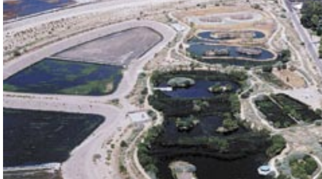
Sweetwater Recharge Facility, City of Tucson. Photo: Bruce Prior, Tucson Water.
