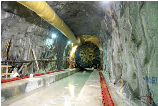
Seven years ago, construction began on the “third straw,” an $817 million water intake that will allow Las Vegas to keep pace with sinking water levels in Lake Mead. The project is scheduled to go into operation this summer.
