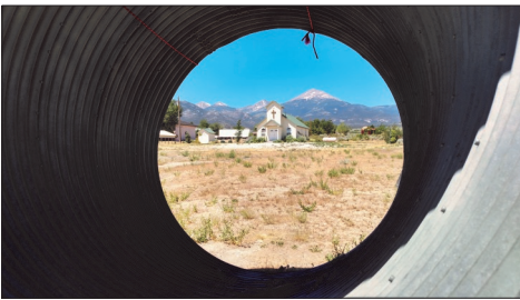
Thanks to Nevada Rangeland Resource Commission for new signs for the 84" diameter pipe in Baker. View from inside.
